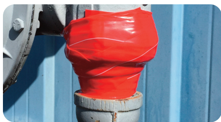
A leaking riser stopped with LLFA Tape
