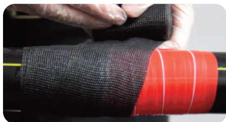
Fiber Armour reinforced squeeze-off
