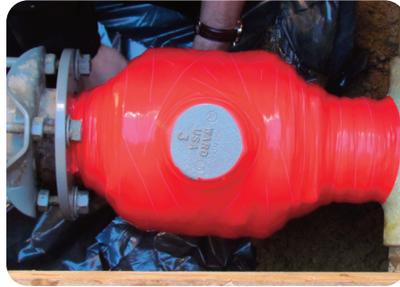
Then wrapped with LLFA Tape
