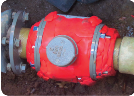
Filled uneven surfaces with LLFA Smooth
