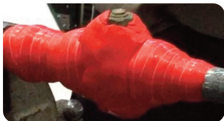
Corroded valve wrapped in LLFA Smooth
