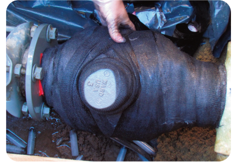
Finished with a layer of Fiber Armour
