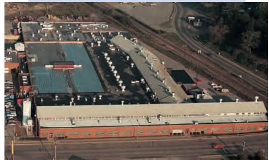
Sensus Metering Systems' headquarters in DuBois, Pennsylvania
